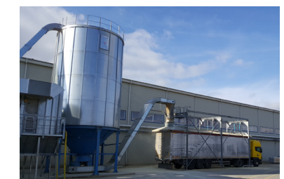
Conveyor, silo and truck loader
